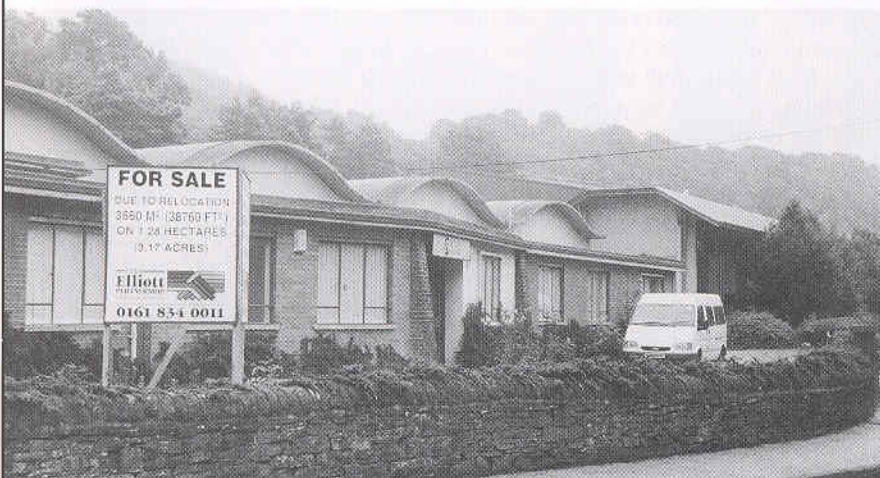
The Eric Britton factory site in Kerridge, now unoccupied, the subject of a recent planning application for residential homes.
